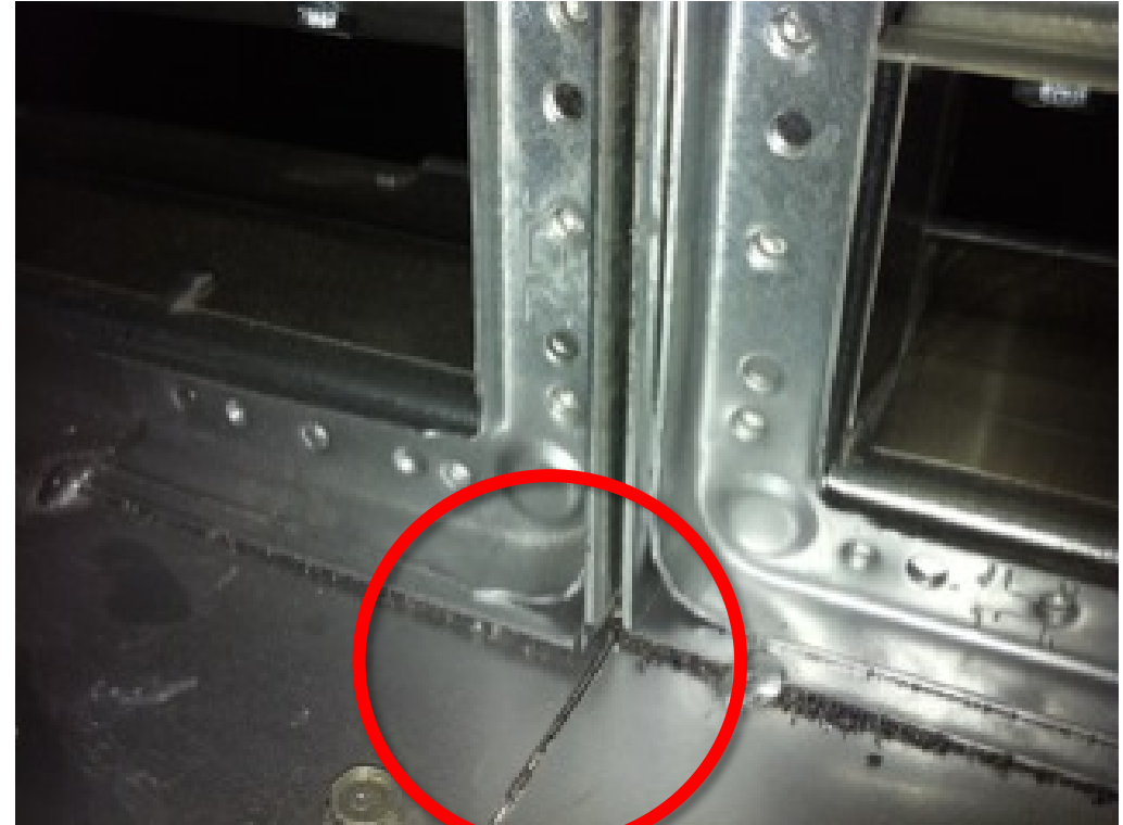
Resizing Damper in the Field
